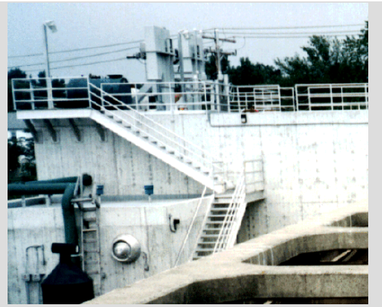
The aerated grit chamber needs to be hosed down
